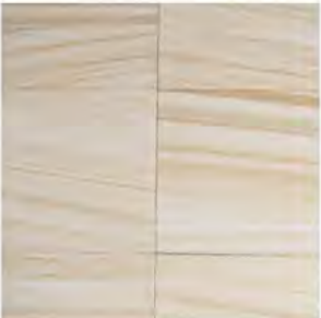
SANDSTONE FACED WALL
