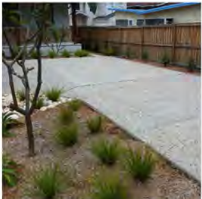
GRIT BLAST COLOURED CONCRETE WITH MARANGA- ROO AND BASSALT AGGREGATE
