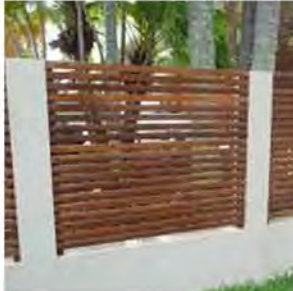
RENDERED WALL WITH TIMBER SLATTS (F4)
